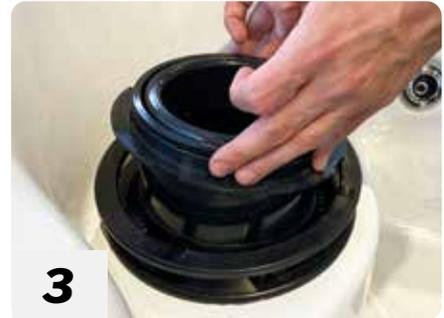
**3** Remove the filter basket and core to reveal the inner weir skimmer box.
