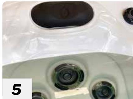
**5** Fill until the water line meets the minimum water level line as indicated by the sticker. Ensure water level does not drop below the skimmer.
