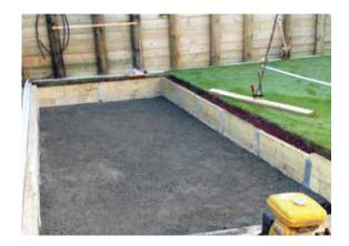
2. Drainage of the pit needs to be fitted. A full length drain should be used that either gravity drains to the outside of the pit, or drains into a sump.
