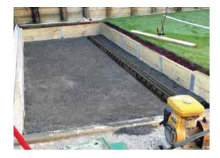
**3.** A reinforced concrete pad should be poured as a foundation.
